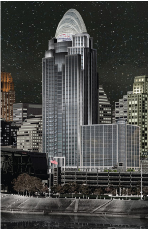
(Above): The Great American Insurance Building at Queen City Square will redefine Cincinnati's skyline with its 40 stories and dramatic tiara.
